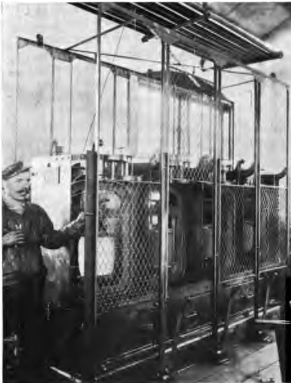
Fig. 3. Sectional Counterweighted Guards which slide vertically.*
